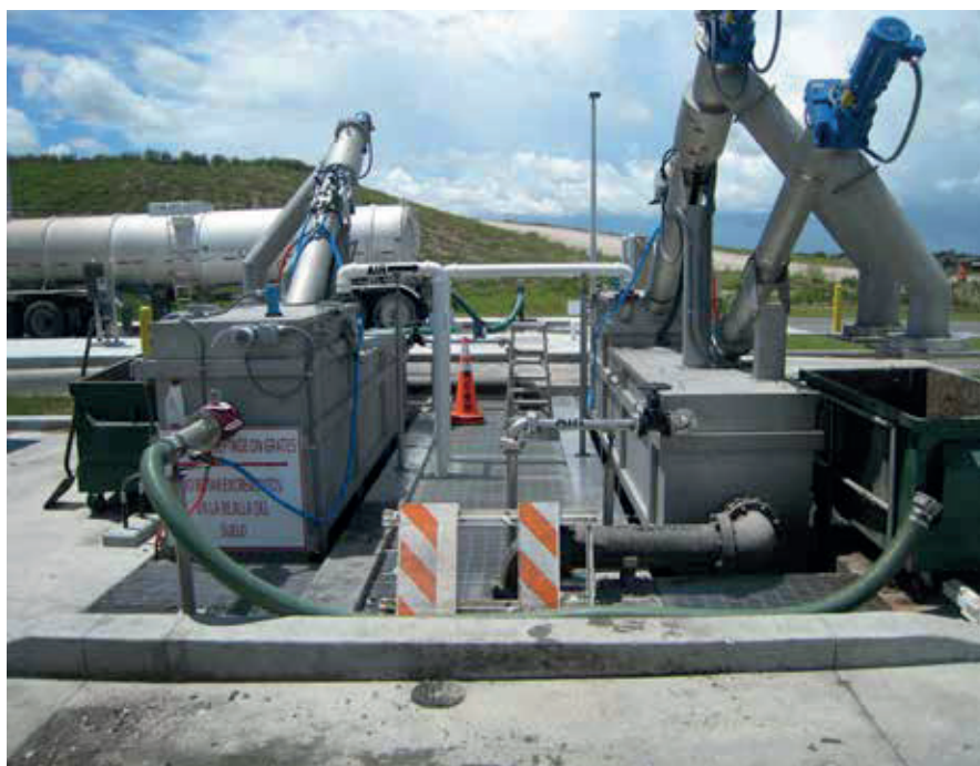
The rotating rake teeth of Lakeside Equipment Corp. (Bartlett, Ill.) Raptor® fine screen fully penetrates the cylindrical screen bars to prevent plugging and blinding. Indian River County and Lakeside Equipment Corp. (Bartlett, Ill.)
