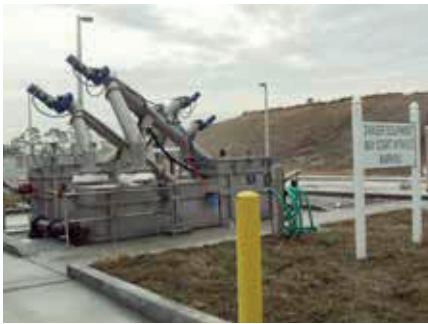
Lakeside's combined screen and grit removal system has been operating at Indian River County Residuals Dewatering Facility for 10 years and is going strong. Indian River County and Lakeside Equipment Corp.
