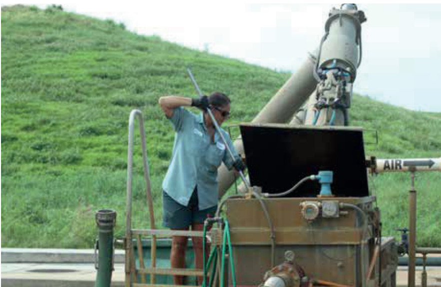
System maintenance requires only a less than 1 h/d cleaning by Indian River County's mechanics who open the system to clean it with a hose. Indian River County and Lakeside Equipment Corp.
